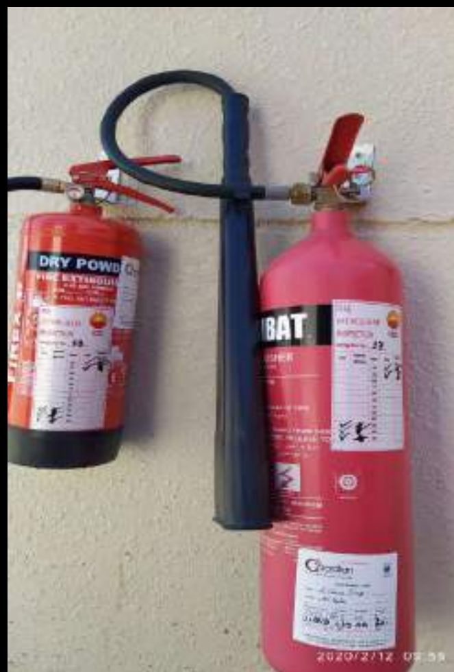
Fire Extinguishers kept wall mounted.
